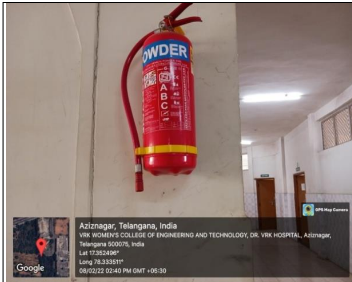
PORTABLE FIRE EXTINGUISHER MOUNTED ON WALL
